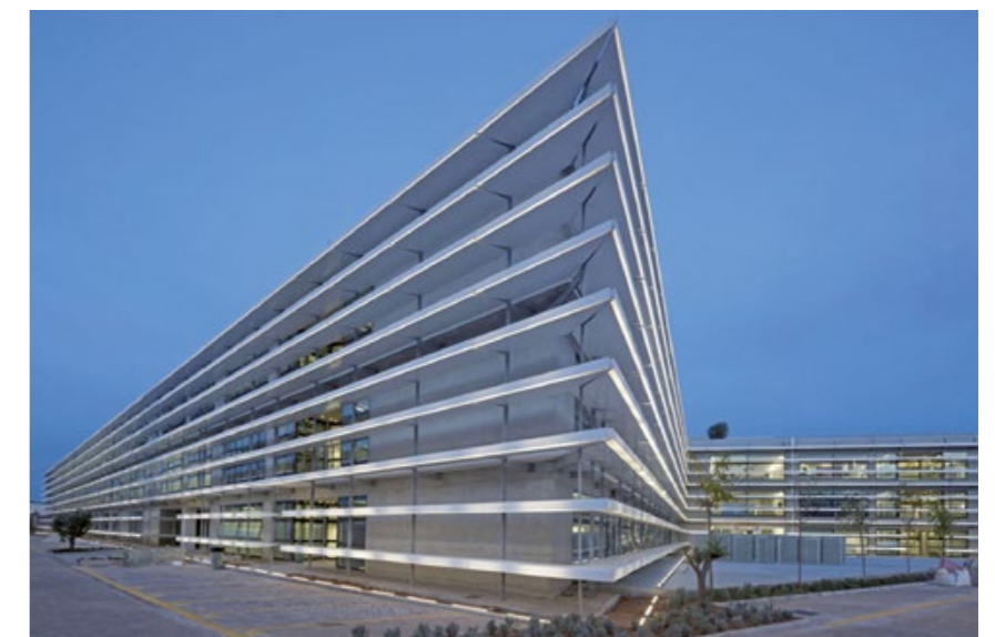
Cosmote head quarter, Karela Office Park · Paiania, Greece The first building in Greece to be awarded the Gold Level of LEED certification in 2013
